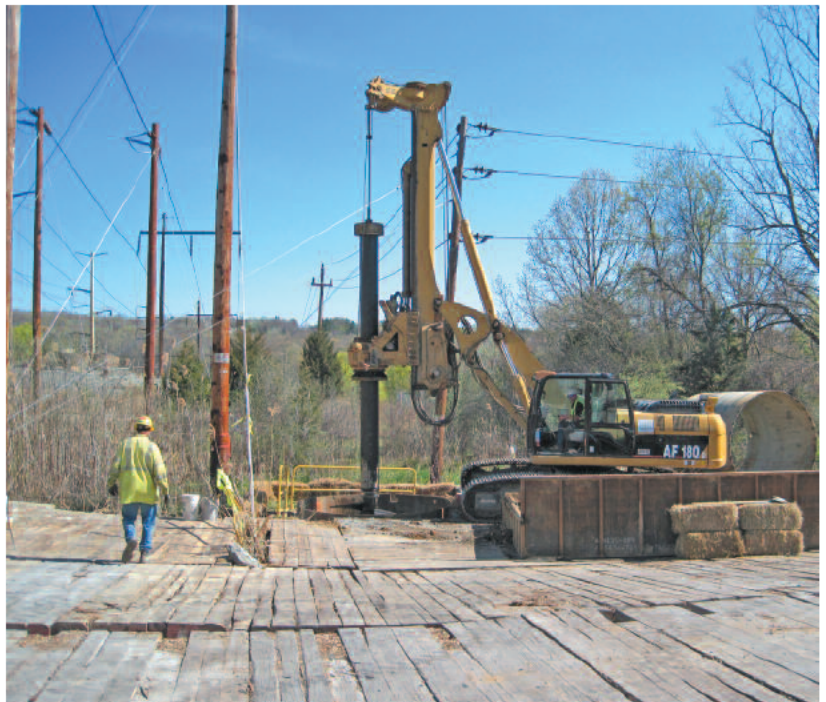
Mats installed to protect sensitive environment.
