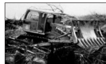
Land Clearing/Site Preparation
