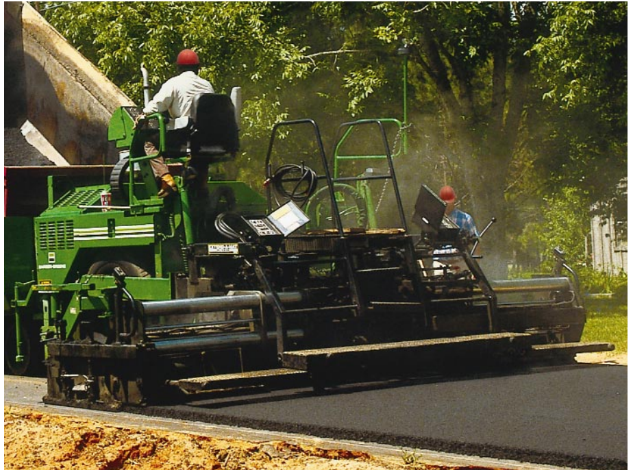
Extend-A-Mat Screed shown with BG-230 Asphalt Paver.
