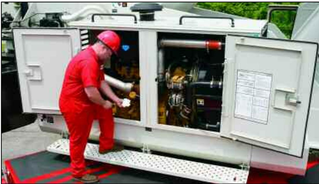
↑ Swing-out doors provide exceptional access to engine components.
